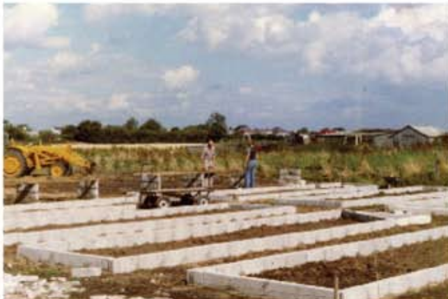
The foundations for the present shop
